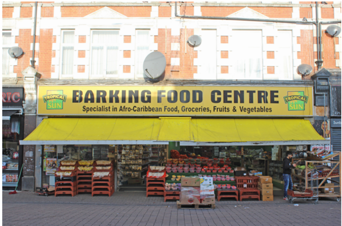
This shopfront has been extended across two historic units with the pilaster and corbel which would have separated them lost. The frontage also has inappropriate internally lit fascia signage and a poorly positioned and dilapidated canopy.
