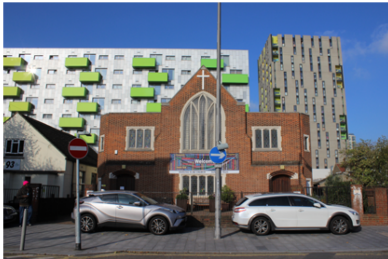
Barking Elim Pentecostal Church in Axe Street is a locally listed building.
