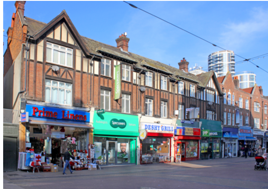
Typical three-storey terraced buildings along East Street.
