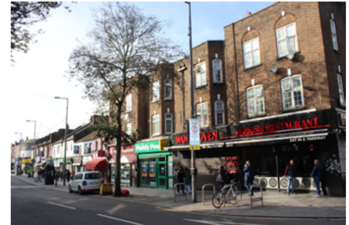
Row of positive buildings, 1-27 Station Parade.
