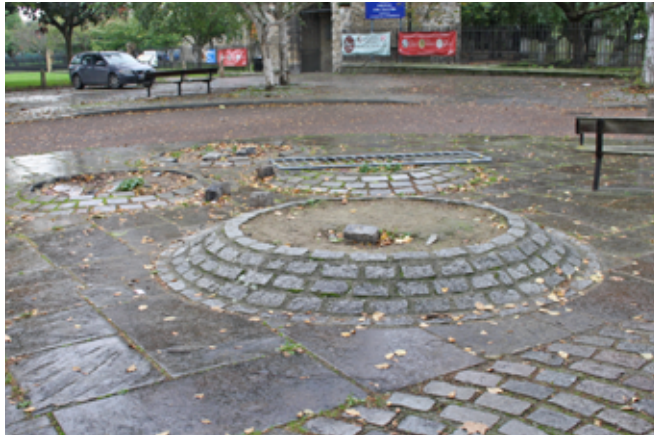
Damage to the granite setts in front of the Curfew Tower and loss of the feature trees.
