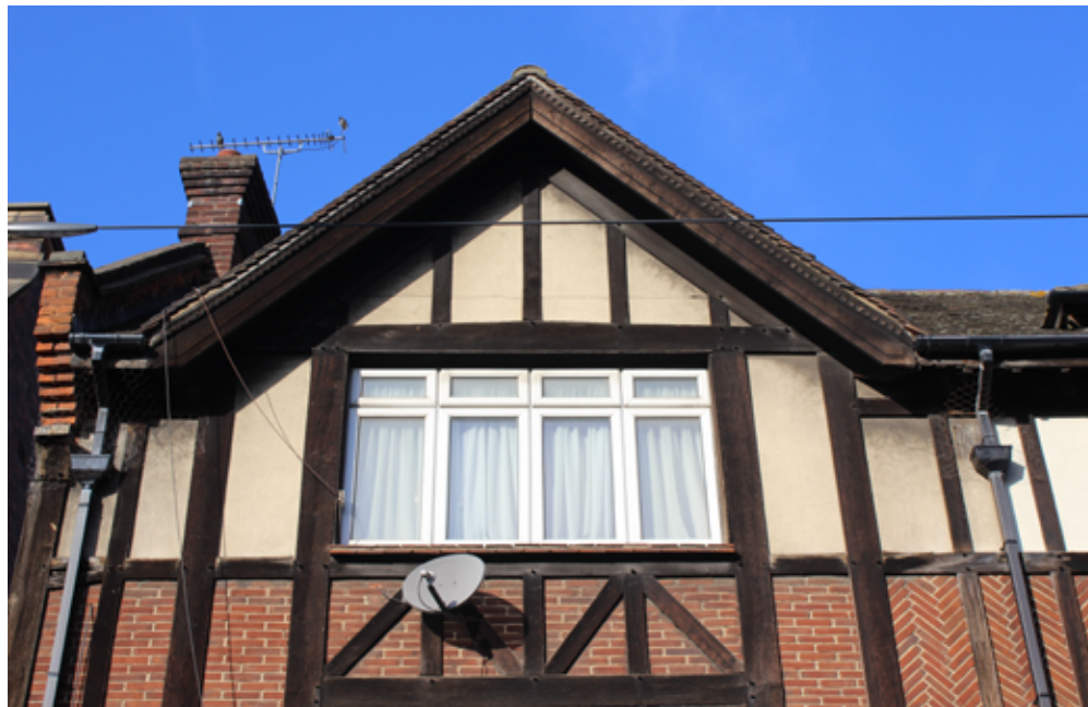
In insensitive replacement of traditional windows with uPVC units is harming the appearance of the conservation area.
