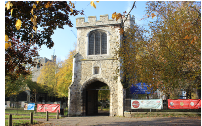
Curfew Tower, Barking Abbey (Grade II*).
