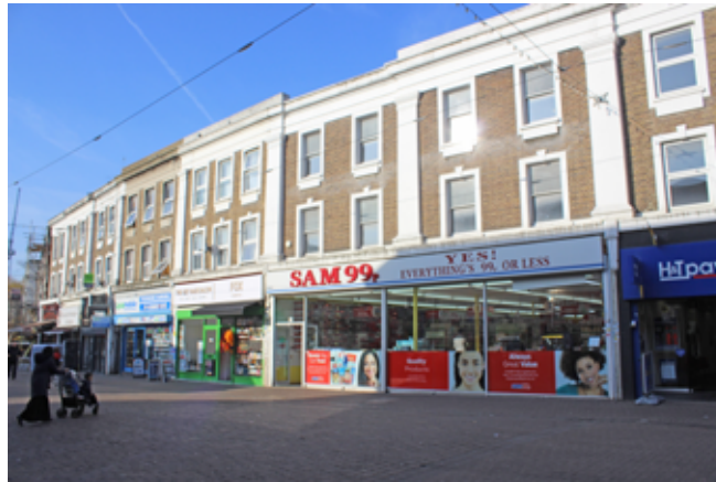
Three storeys terraced buildings on the north side of East Street.
