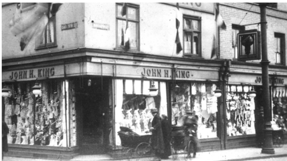
This Victorian shopfront (John H. King) on the corner between East Street and the Broadway shows the building in place before the 1930s 2a-4a East Street (former Burtons). (Barking & Dagenham Archives and Local Studies, Valence House: HHL2621)
