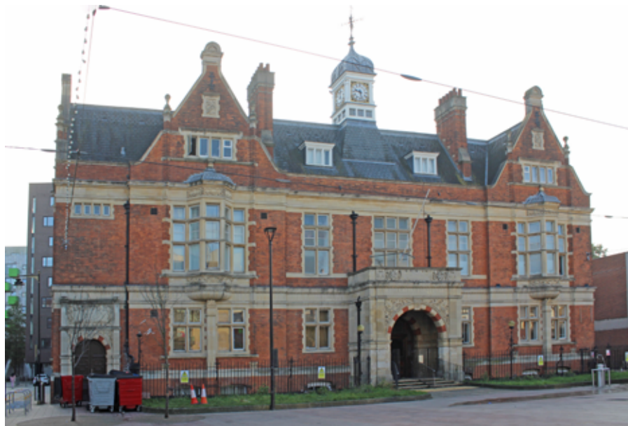
Barking Magistrates' Court is a landmark building for its highly decorative appearance and position at the heart of East Street.
