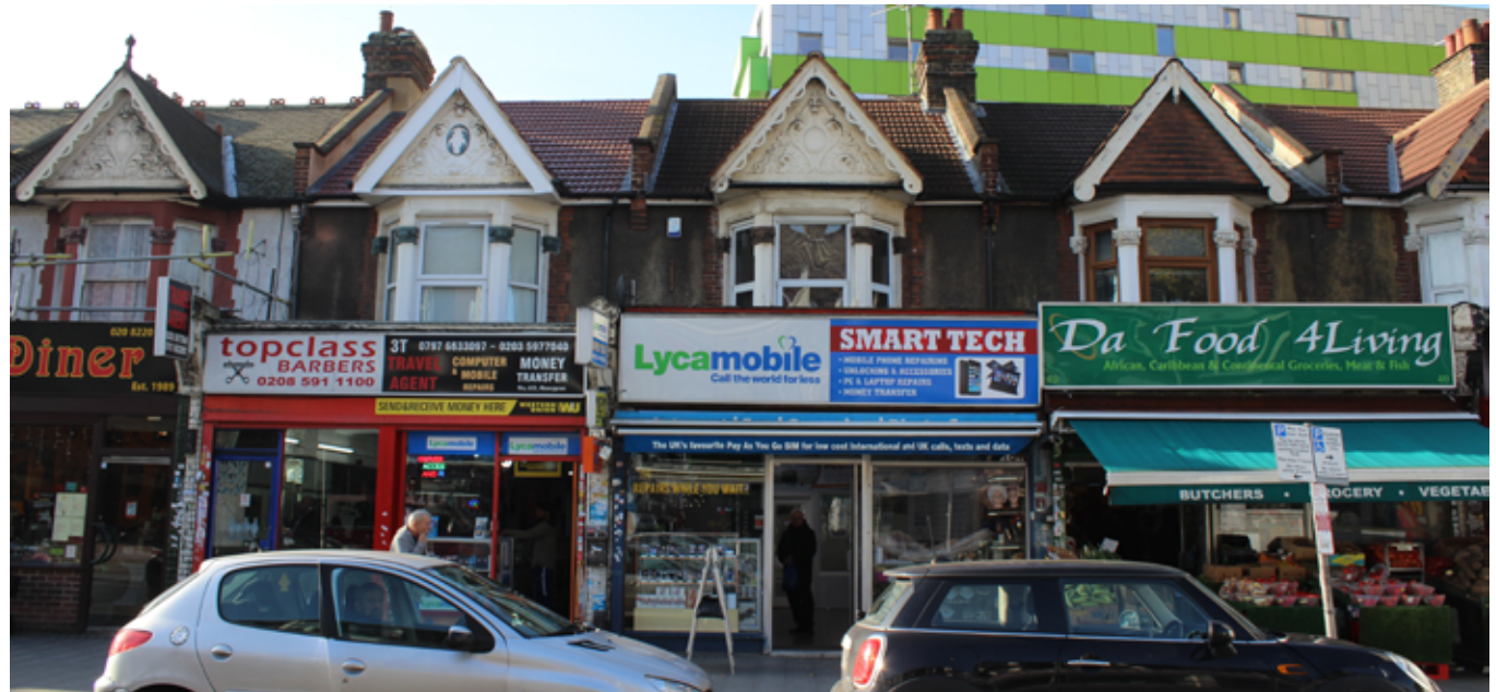
Nos. 40-46 Ripple Road are positive buildings, despite later insensitive modern shop fronts and signage
