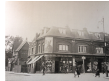
East Street/Ripple Road junction showing 1a Station Parade with an active frontage and windows on the upper floors, which are covered today by an unnecessary superficial render (see photo on p.26)
